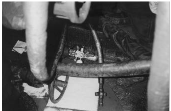
Fig. 5-Remote-fire gun connected to wellhead.
