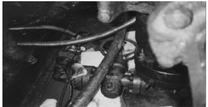
Fig. 4-Remote-fire gun connected to wellhead.
