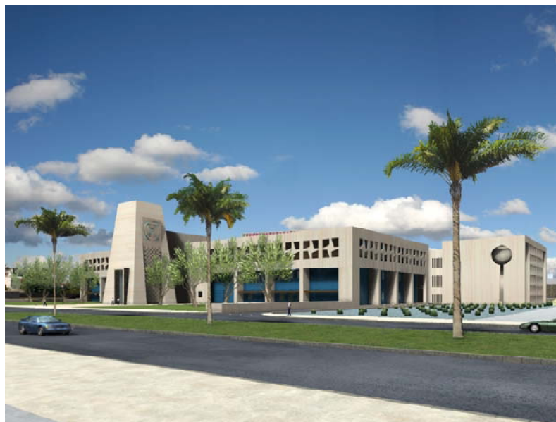
Fig. 7—Engineering building now under construction on the campus of TAMU—Q.
